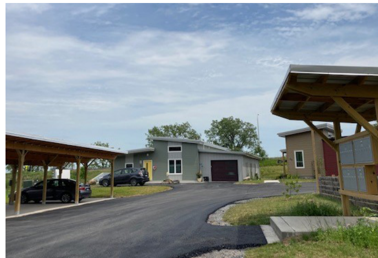
Photo: Lake Tunnel Solar Village
