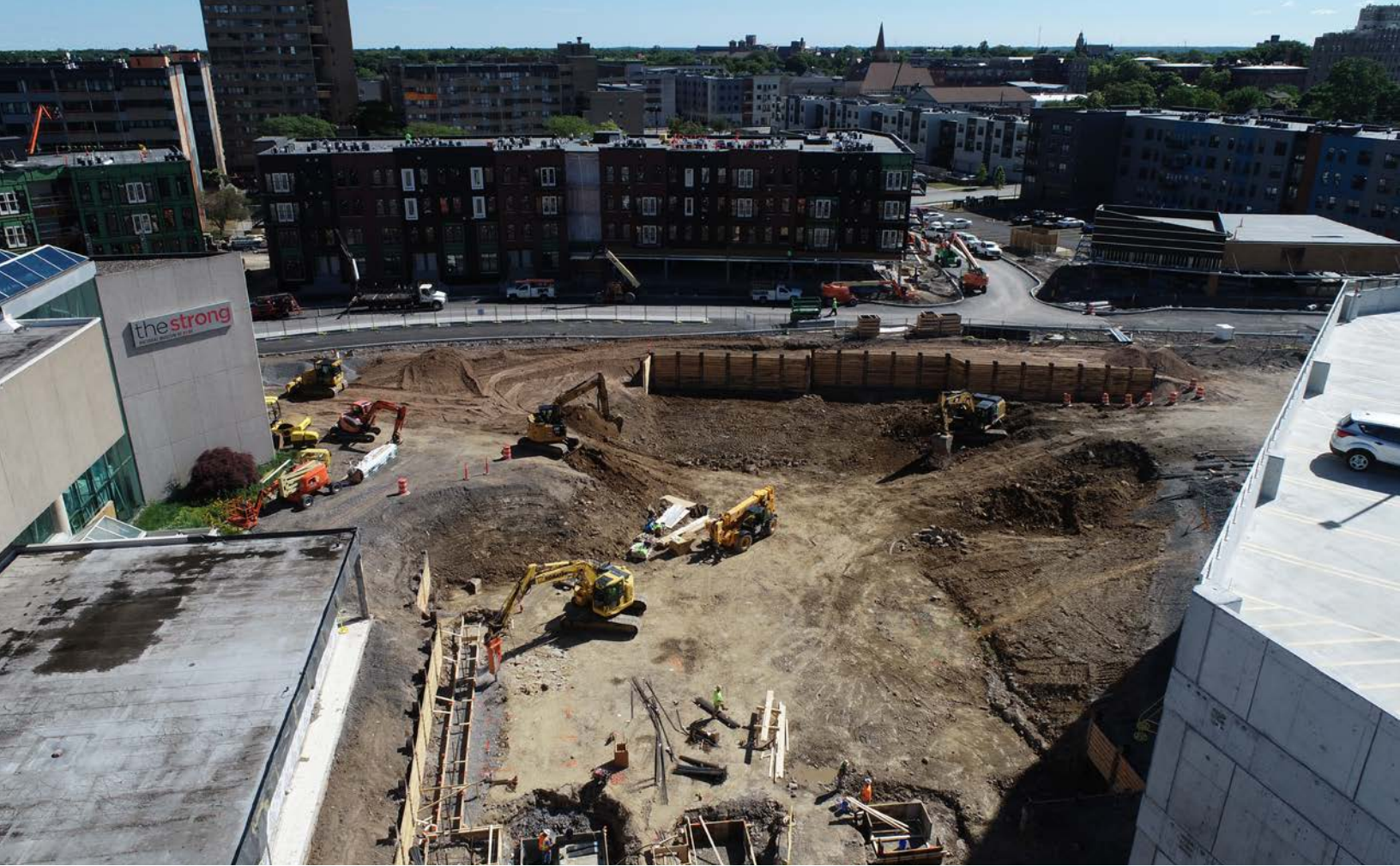
Photo: Construction at The Strong Museum expansion and Neighborhood of Play
