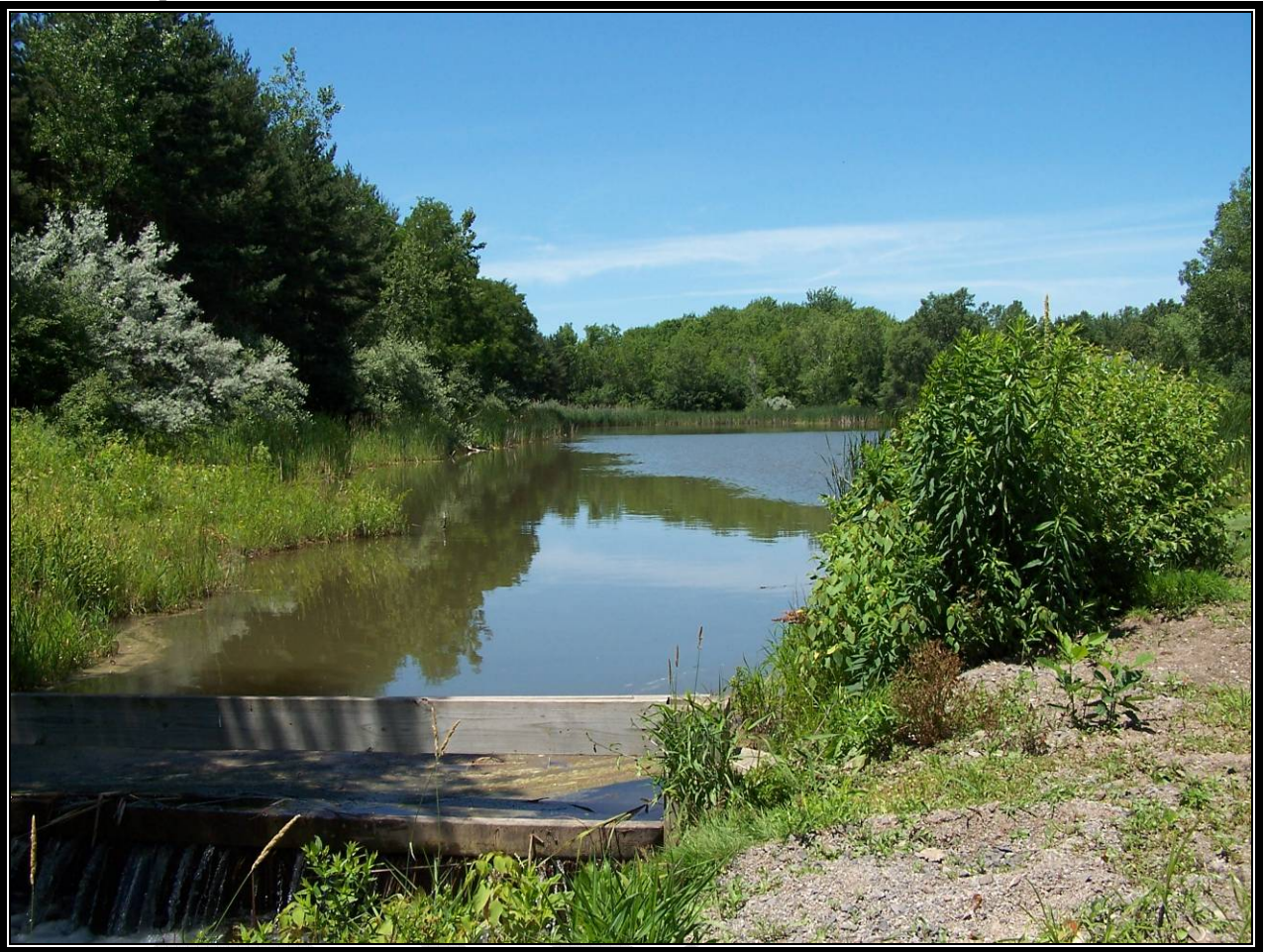
Figure 6. Hidden Valley Pond Outlet – leaking weir lacking water quality or quantity control.
