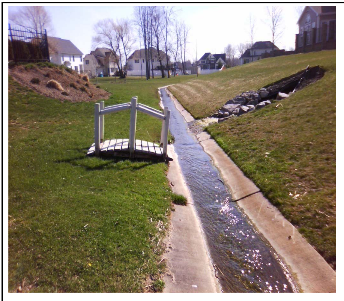
Figure 15: Channelized Stream Segment in Subwatershed E with Severity Score of 5
