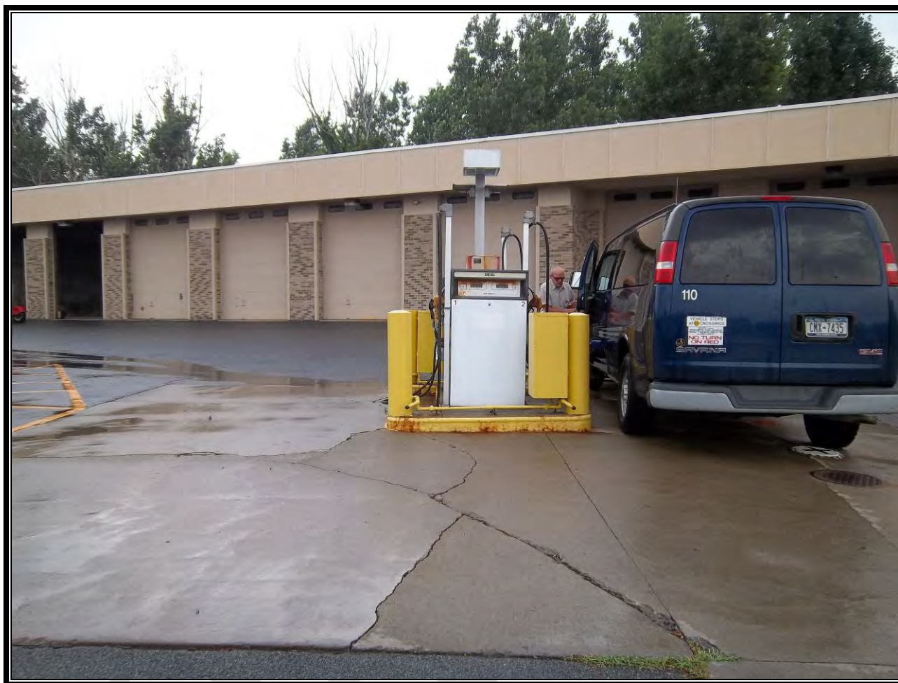
Figure 17. An example of a potential watershed Hotspot in Buckland Creek – an uncovered fueling station
