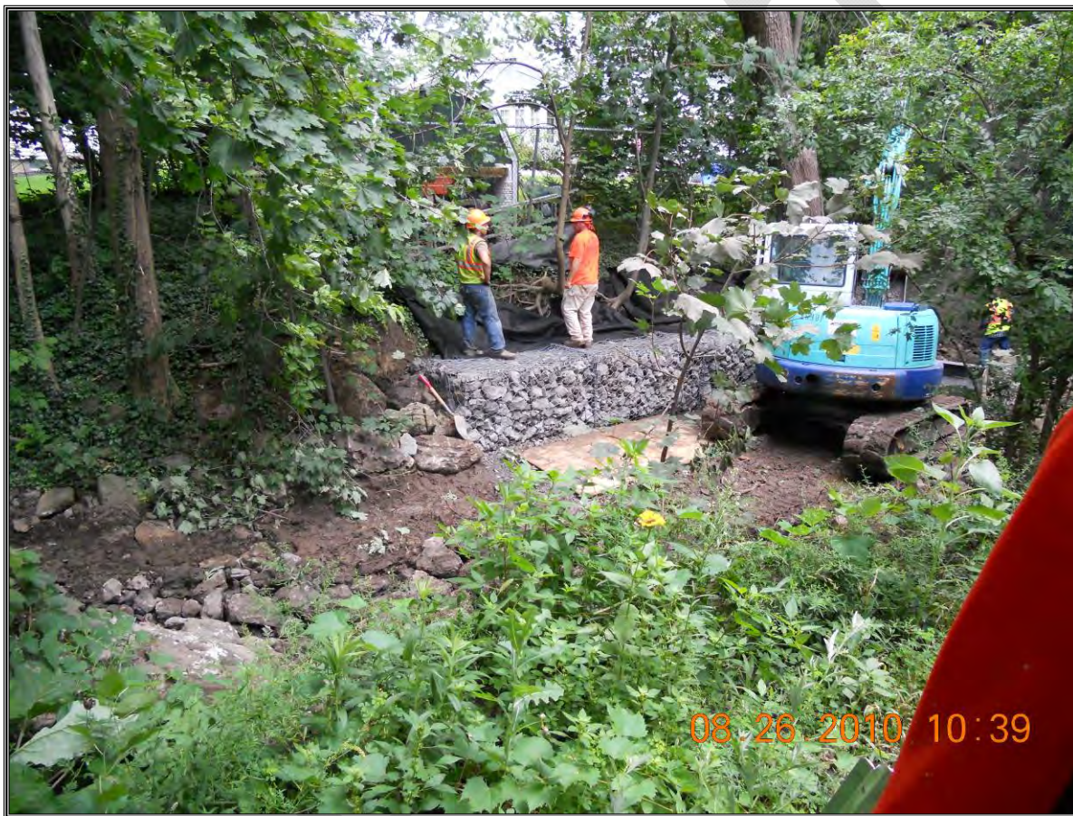
Figure 14. Stream Bank Erosion site being stabilized with rock-filled gabion baskets
