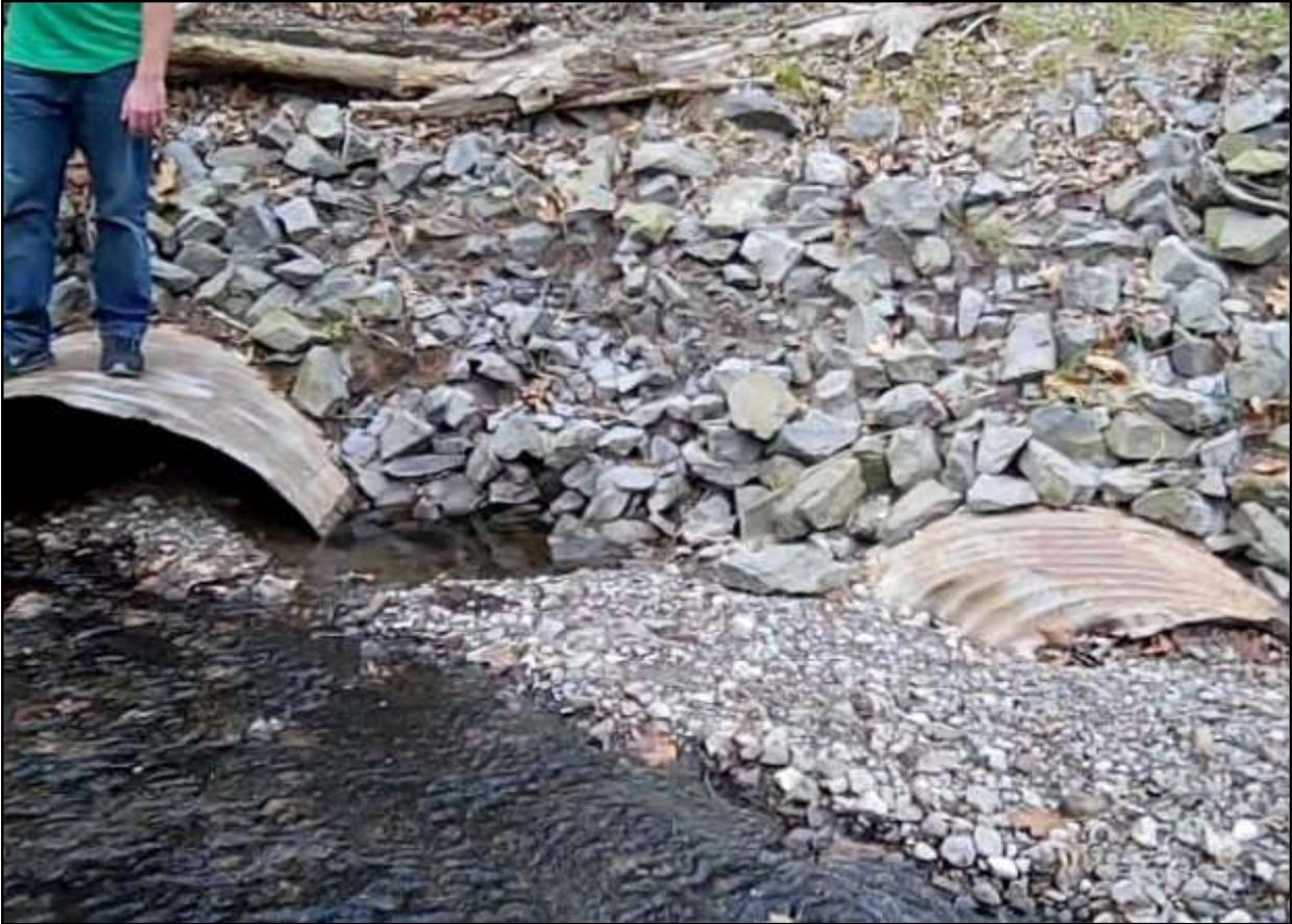
Figure 5. Upstream erosion of glacially laid gravels regular deposit at these twin culvert pipes on South Glen Road, Irondequoit, NY
