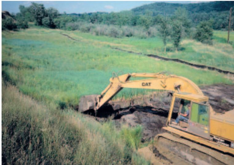
*Salvage marsh surface (SMS) is excavated from the wetland that is to be filled and is stockpiled for application over the created wetland. SMS is a critical element for providing the appropriate hydrological and chemical environment for wetland plant establishment.*
