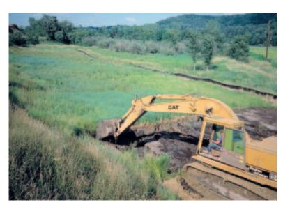
Salvage marsh surface (SMS) is excavated from the wetland that is to be filled and is stockpiled for application over the created wetland. SMS is a critical elementforproviding the appropriate hydrological and chemical environment for wetland plant establishment.
