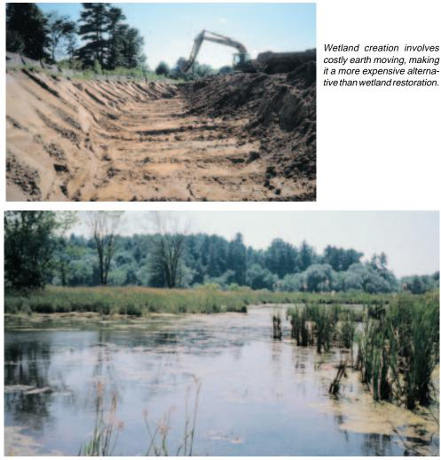
**Figure 5.** The type of wetland targeted for a creation or restoration can have a large effect on the success of the project. The Wisconsin Department of Transportation/U.S. Geological Survey restoration site targeted a shallow-water marsh (a relatively easy wetland type to restore). This resulted in a higher wetland success rate at the restoration site than at the creation site when evaluated as percent of site acreage.
