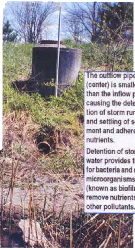
The outflow pipe (center) is smaller than the inflow pipe, causing the detention of storm runoff and settling of sediment and adherent nutrients. Detention of stormwater provides time for bacteria and other microorganisms (known as biofilm) to remove nutrients and other pollutants.
