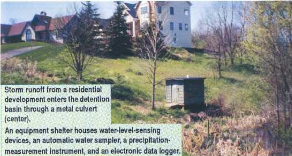
Storm runoff from a residential development enters the detention basin through a metal culvert (center).
