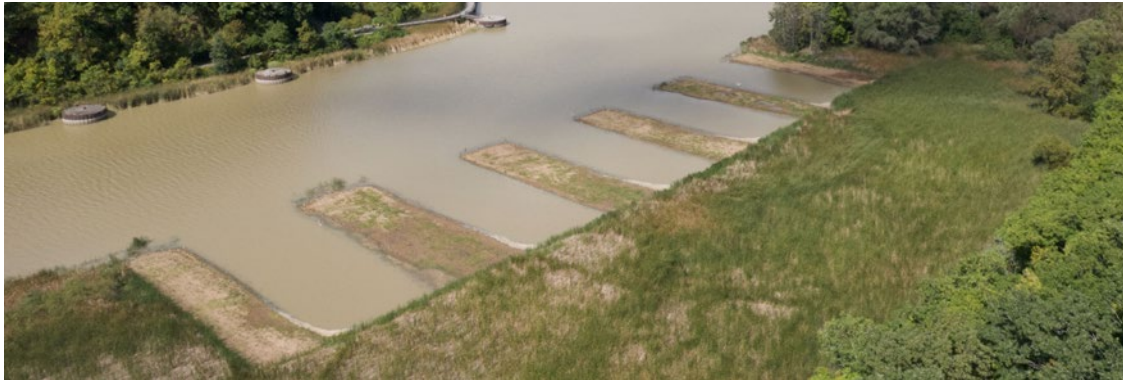
Figure 9: Completed Wetland C North site
