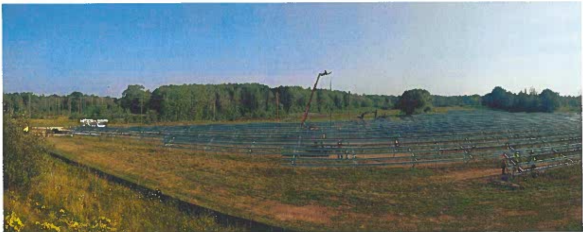
Photo 5. Solar facility under construction on Miller Road in Henrietta, 2018.
