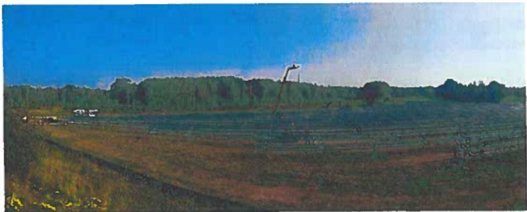
Photo 5. Solar facility under construction on Miller Road in Henrietta, 2019.
