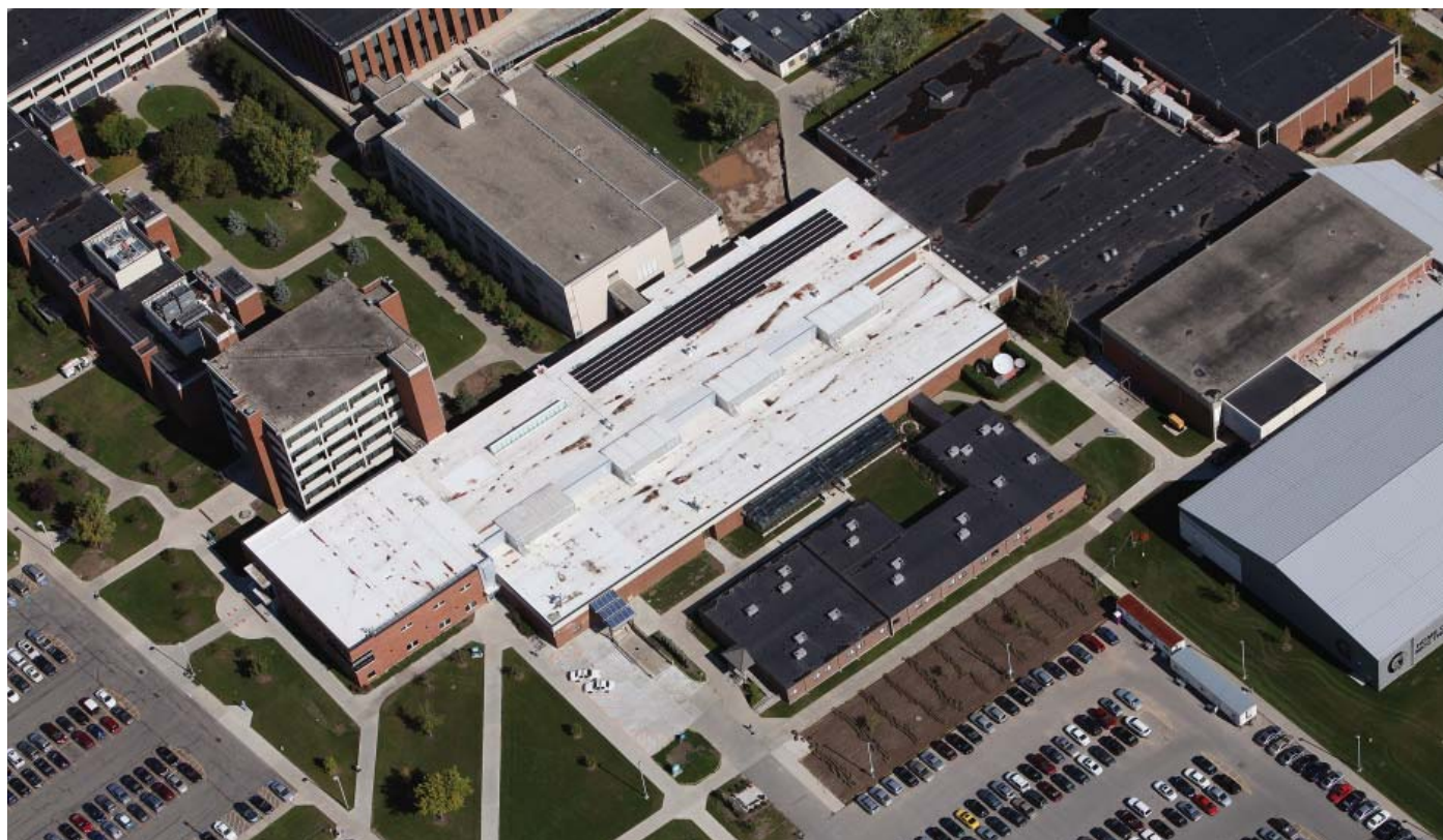
AERIAL - WHITE ROOF/SOLAR PANELS
