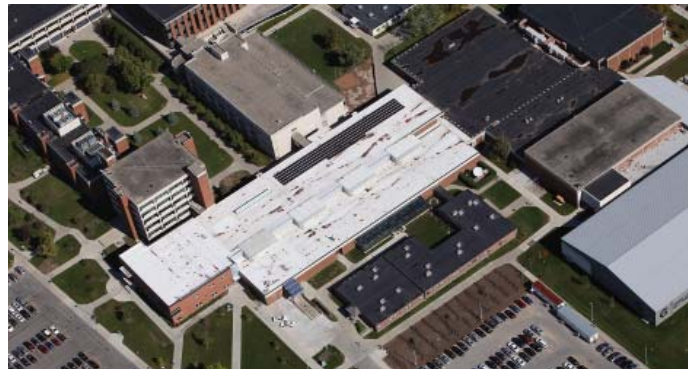
AERIAL - HIGH ALBEDO ROOF + PHOTOVOLTAICS FIGURE 2.1
