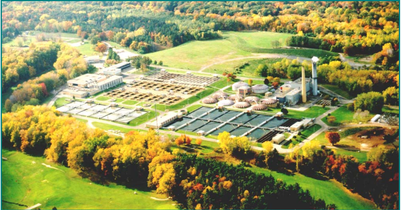
An aerial view of the Frank E. VanLare Wastewater Treatment Facility
