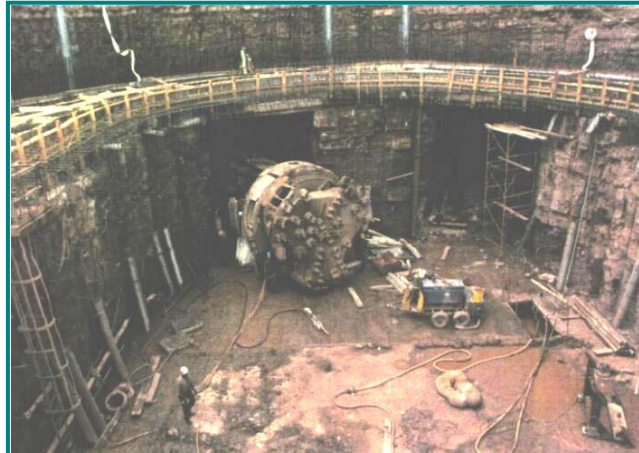
The head of a mole (showing its teeth) emerges from a tunnel.
