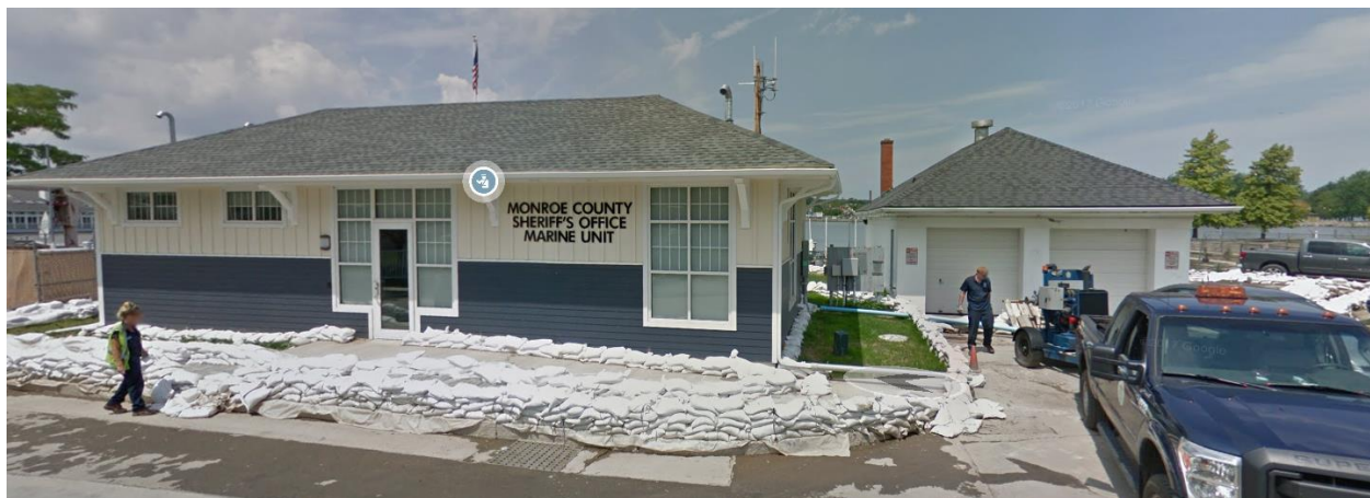
Sand bags surround the Monroe County Sherriff's Office Marine Unit to protect from damage during the 2017 lake flooding event. Source: Google StreetView
